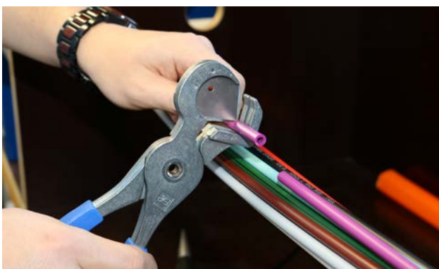
5. Cut off another 3 to 4 cm to create enough space for the connector and end stop.
