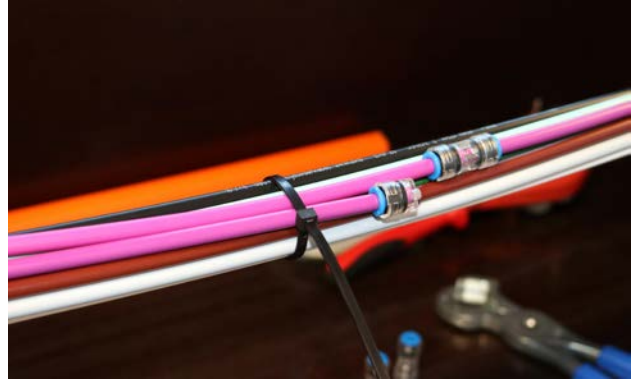
8. Fasten the connection and end stopper with cable tie or the like.
