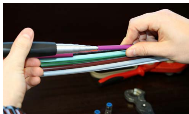
6. Reroound the interfaces using the 5/20 tool.
