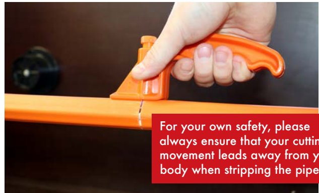
2. Use the sheathing knife to prick the sheathing at the notch and push it as far as to the 2 nd notch.
