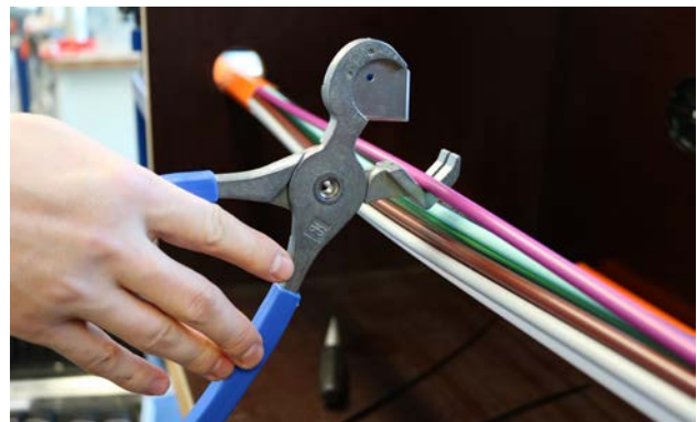
4. Perform a perpendicular cut on the pipe to be cut using the pipe cutter.
