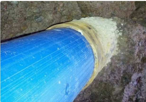
Geringe Querschnittsreduzierung – Close-Fit Low reduction of the cross-section – Close fit
