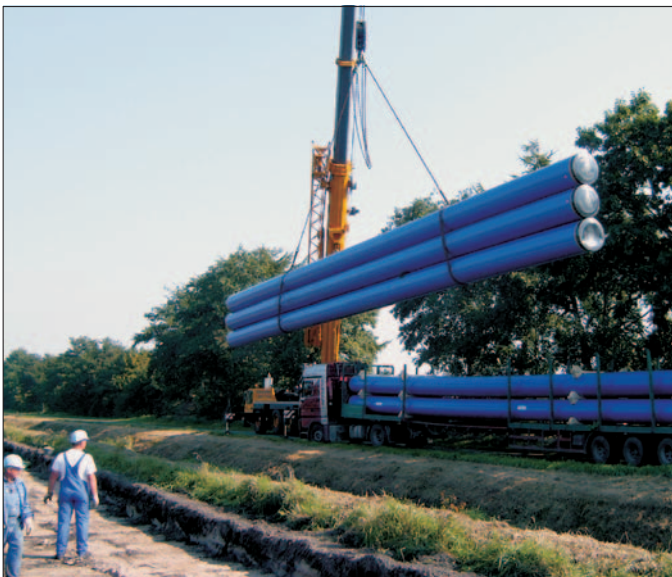
Fig. 4: Delivery of the 22 m HDPE pipes
