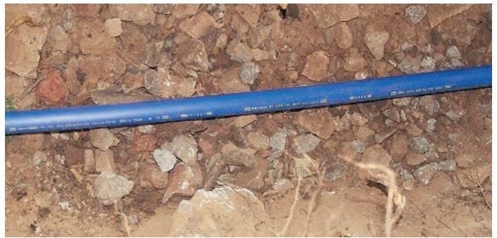
Fig. 5: Alternative (sandless) installation of a pipe
