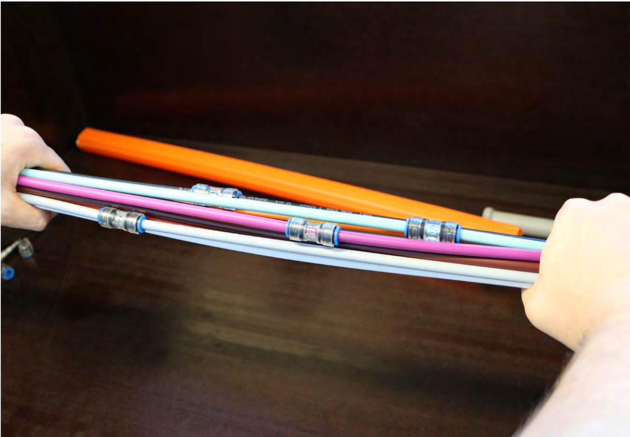
7. Slide the connector and end stopper on up to the stop. Connect the house connection pipe.
