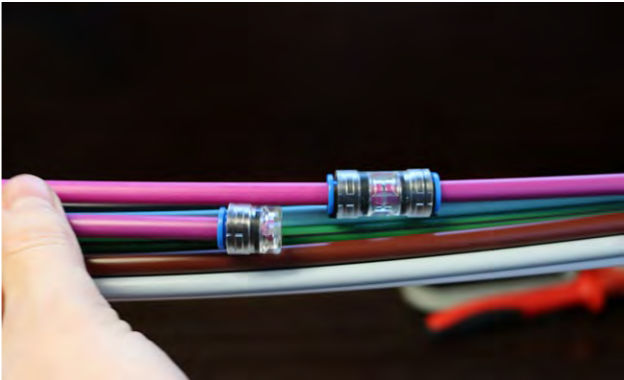
7. Slide the connector and end stopper on up to the stop. Connect the house connection pipe.
