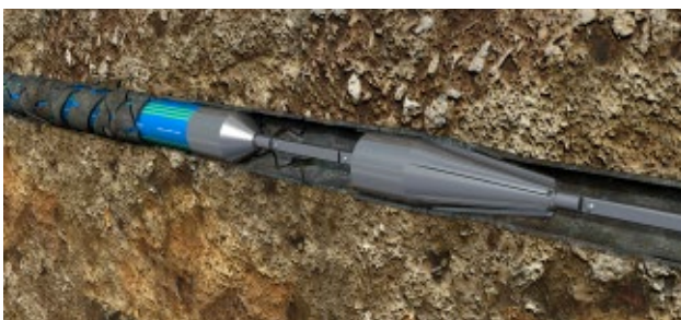
Fig. 11: Dynamic pipe bursting (pipe cracking)
