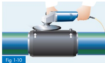
Fig 1-10 Removal of the contact plugs
