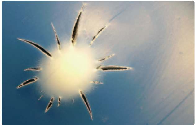
Fig 2-21: Stress crack on the inside of the pipe caused by point load and incorrect choice of material (source: HESSEL technical engineering)
