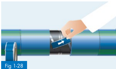
Fig 1-28 Restoring the electrical connection
