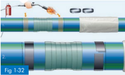
Fig 1-32 Preheating the pipe surface and applying the hot-melt adhesive
