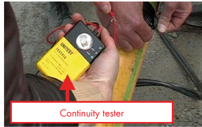
Fig 1-58: Verification of integrity using a continuity tester
