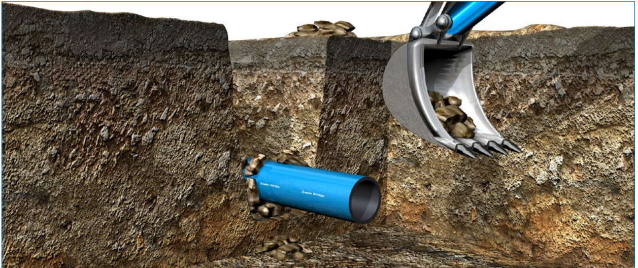
Fig. 4: The use of pipelines with integrated protective layers is recommended when dispensing with a sand bed.
