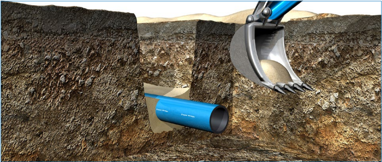
Fig. 3: Standard pipes are installed in a sand bed
