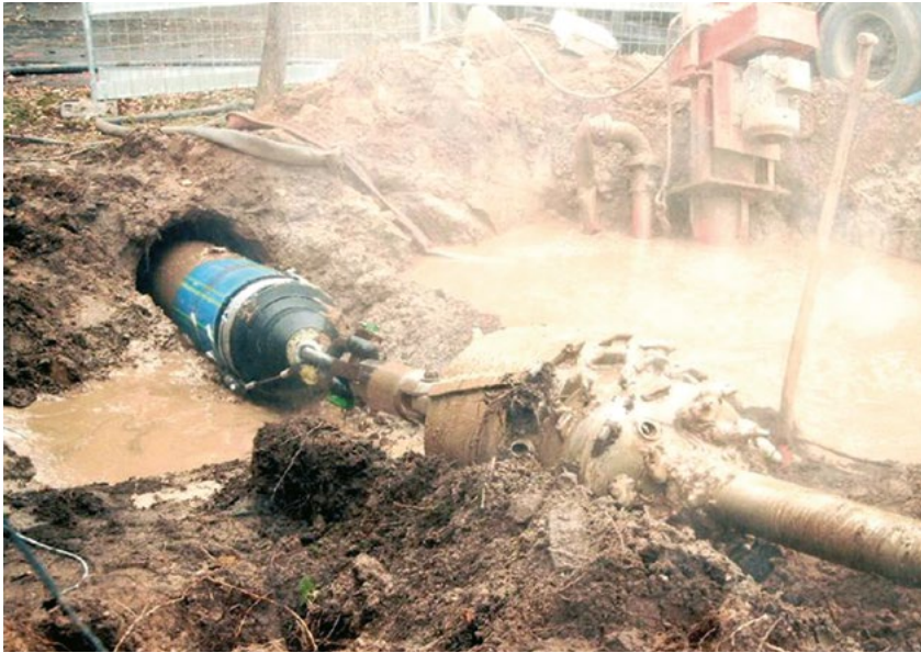
Fig. 30: Pipe with additional protective layer after the insertion process
