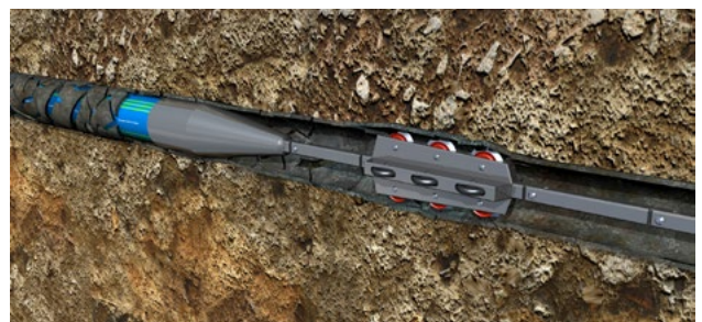
Fig. 12: Static pipe bursting
