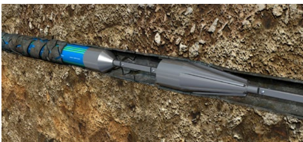
Fig. 11: Dynamic pipe bursting (pipe cracking)
