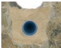
open trench installation in sandbed
