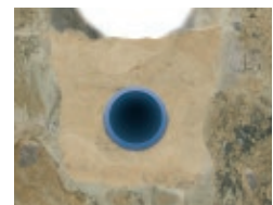
open trench installation in sandbed
