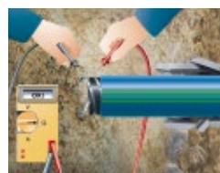
Integrity test after trenchless installation
