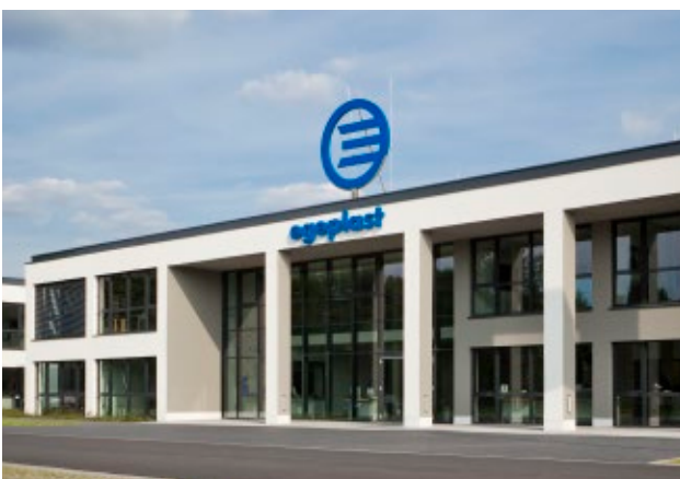
Head Office and production location is Greven/Germany
