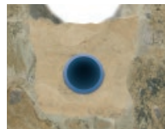
open trench installation in sandbed
